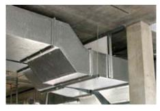
**Ducting for Ventilation and Smoke Extract** Promat DURASTEEL® ducting is commonly used in the London Underground.
